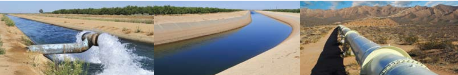
California irrigation canal; pipeline in the Mojave Desert
